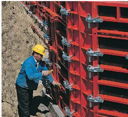
Typical example of modern construction: oblique angles, returns and different wall thicknesses.
