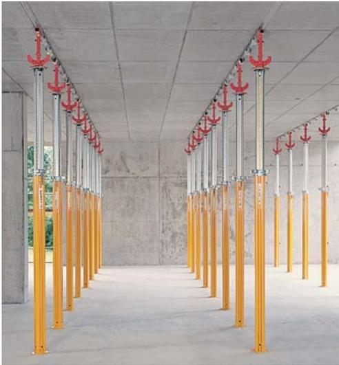
After striking, only the props with dropheads and cover strips remain in place.
