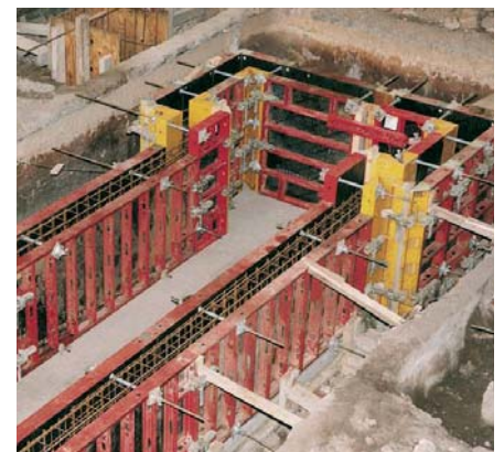
Foundations formed without a crane.
