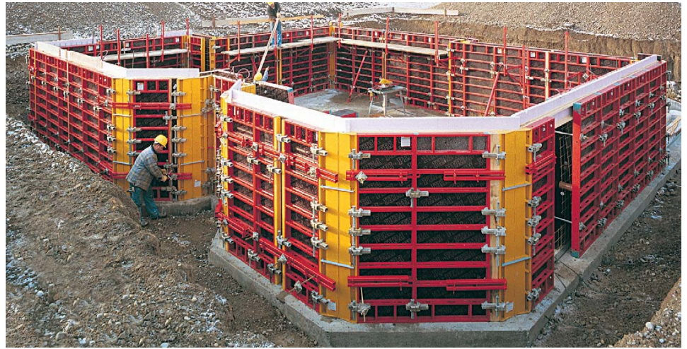
Basement walls formed without a crane using PERI DOMINO.
